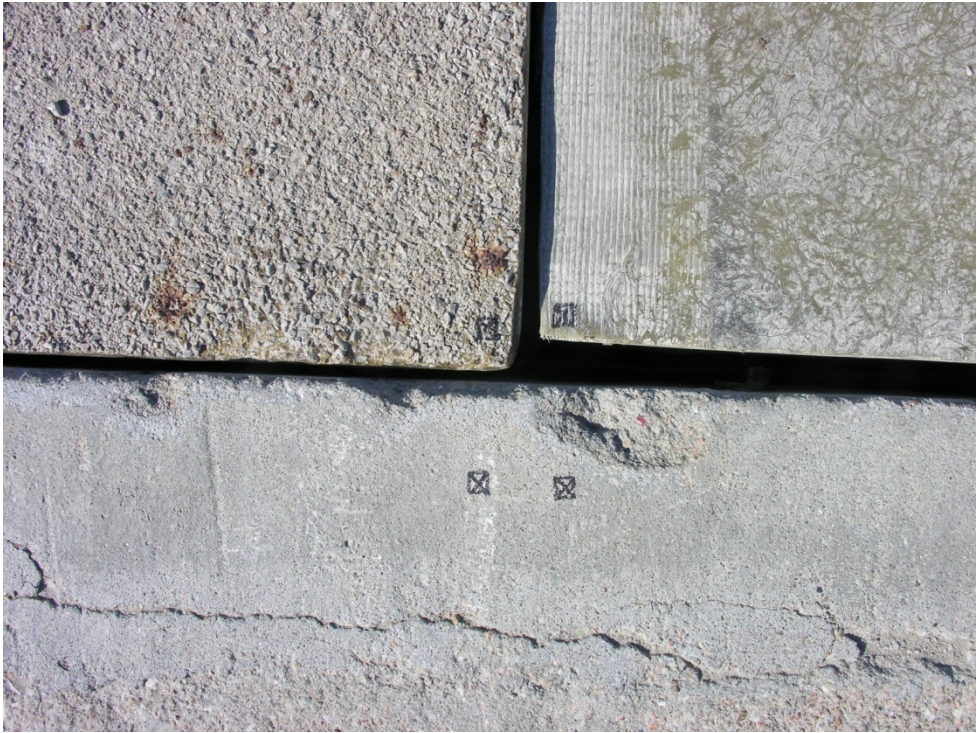
Figure 31. Panel Shift - Joints 3 and 4 (Top) and 4 and 5 (Bottom), Test No. KSFRP-1
